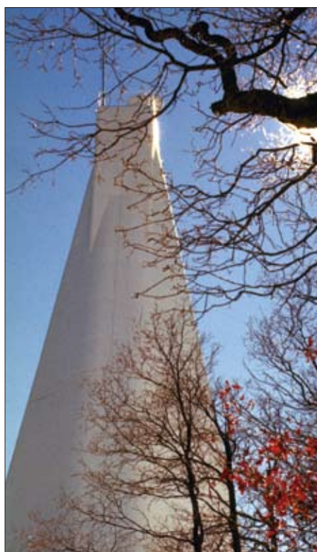
1: ROSA is installed on the Richard B Dunn Solar Telescope (DST) at the National Solar Observatory, Sacramento Peak, New Mexico. Although the tower of the DST rises 41.5 m above ground level, another 67 m of the telescope lies out of sight underground. (NOAO/AURA/NSF)
